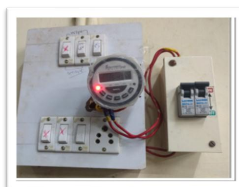
Fig-2 Timer: To maintain 14hrs light and 10hrs Dark Cycle
